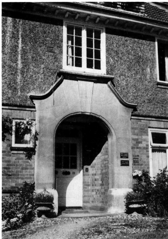
Fig. 20 26 Redlands Road, Reading
